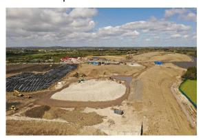
The contractor has already commenced the capping of the site with the Linear Low Density Polyethylene (LLDPE) sheeting.
